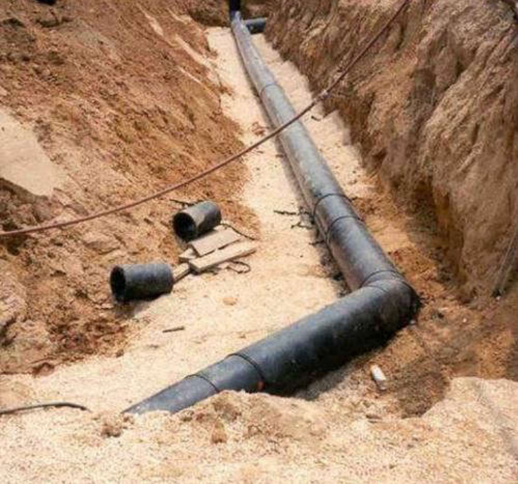
Figure 21: Pipe Placement in Open Trench
