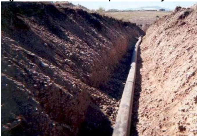
Figure 23: Trench Wall Sloped for Safety
